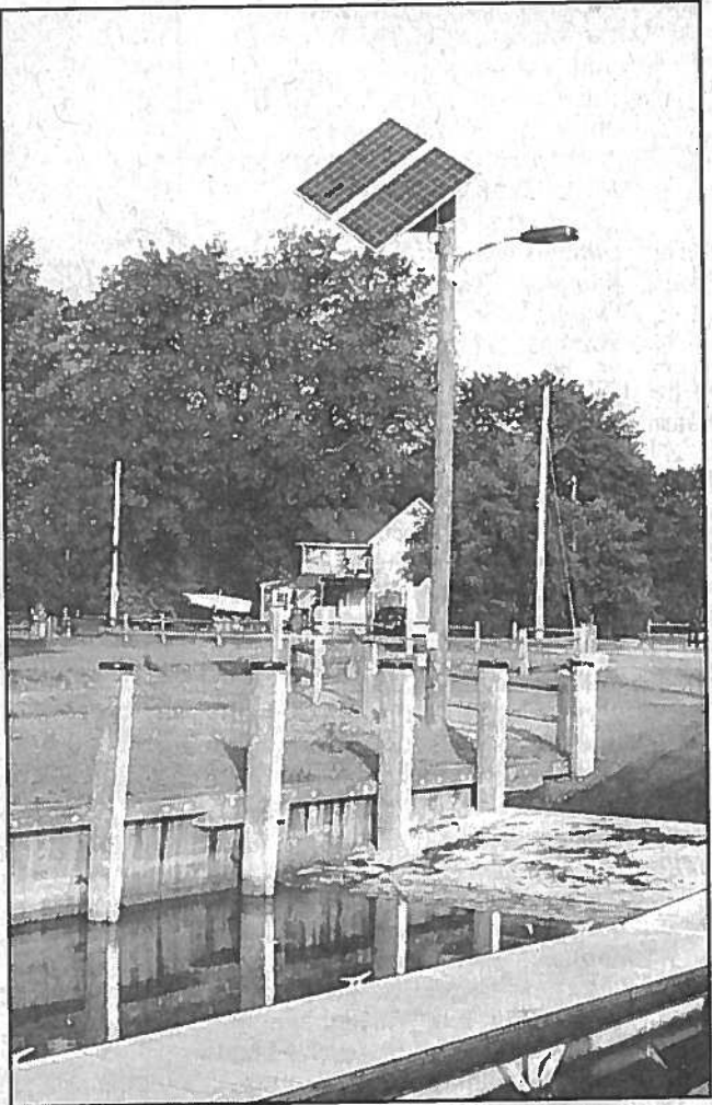
A sun-tracking solar panel was recently installed at Oak Creek Landing to supply power to the parking lot lights as well as to the electric grid.
